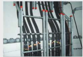
Wind Turbine Tower Internal Piping
