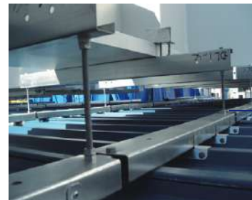
◀ Pier Over Plate Mounting
