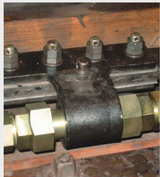
Railroad Switch Moving Portion
