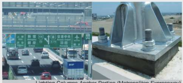
Lighting Columns Anchor Portion (Metropolitan Expressway)
