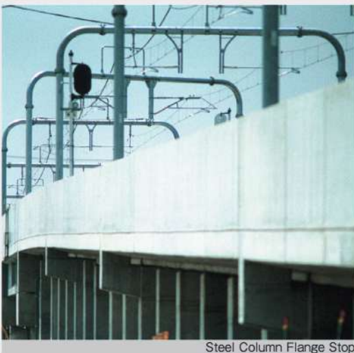
Steel Column Flange Stop
