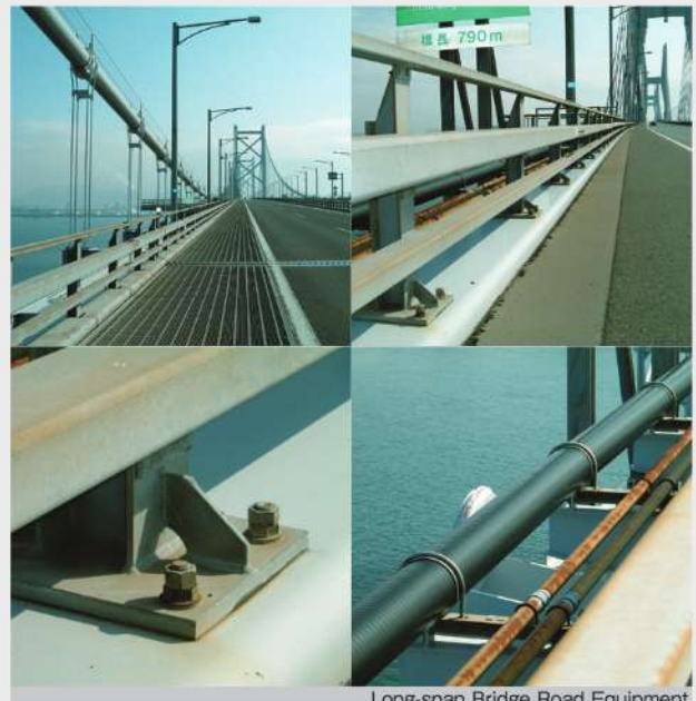
Long-span Bridge Road Equipment
