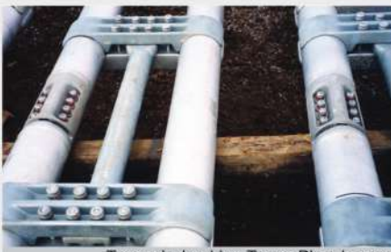
Transmission Line Tower Pipe Jumper
